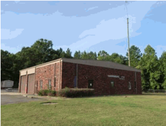
Front & side of building
