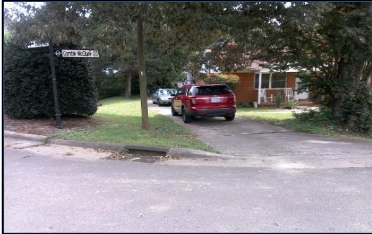
Corner 3 No Ramp (3z)
