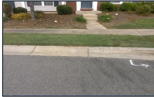
Corner 3 No Ramp (3z)
