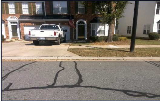
Corner 3 No Ramp (3z)
