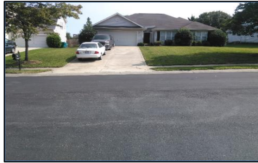
Corner 2 No Ramp (2z)
