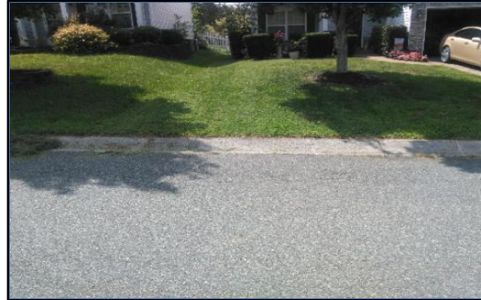
Corner 4 No Ramp (4z)
