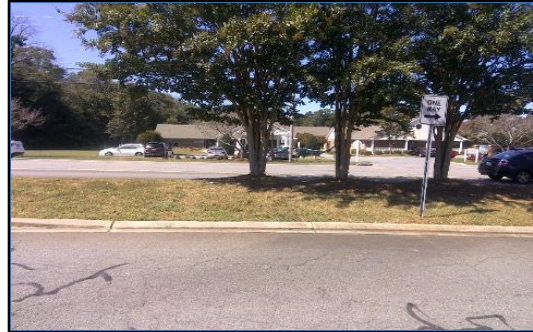
Corner 4 No Ramp (4z)
