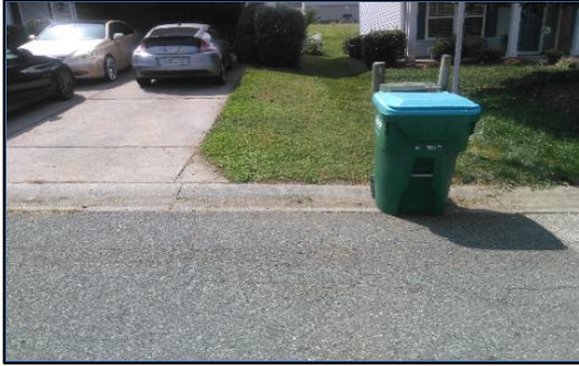
Corner 1 No Ramp (1z)
