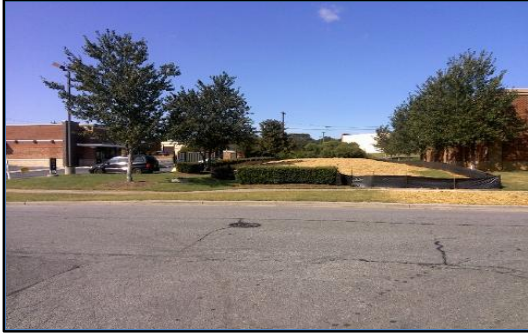
Corner 1 No Ramp (1z)
