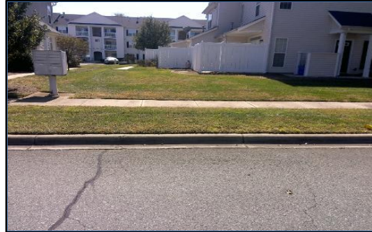
Corner 4 No Ramp (4z)
