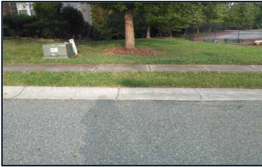
Corner 1 No Ramp (1z)
