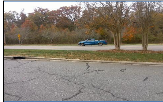
Corner 4 No Ramp (4z)
