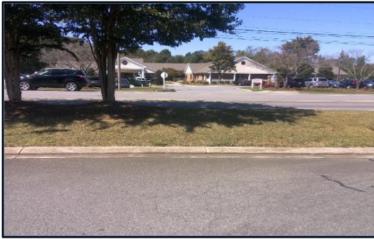
Corner 1 No Ramp (1z)
