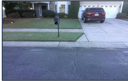
Corner 2 No Ramp (2z)
