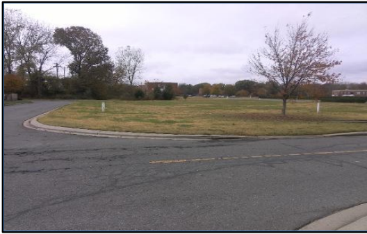
Corner 1 No Ramp (1z)
