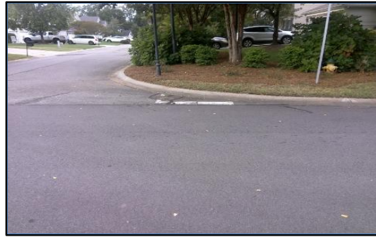
Corner 2 No Ramp (2z)
