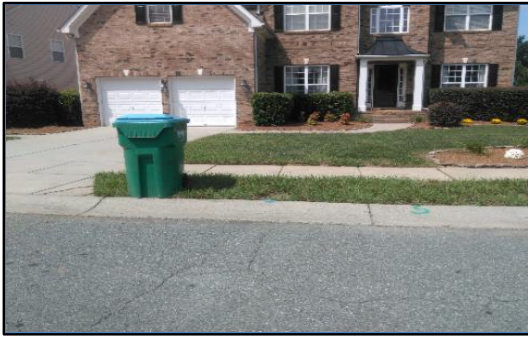
Corner 1 No Ramp (1z)
