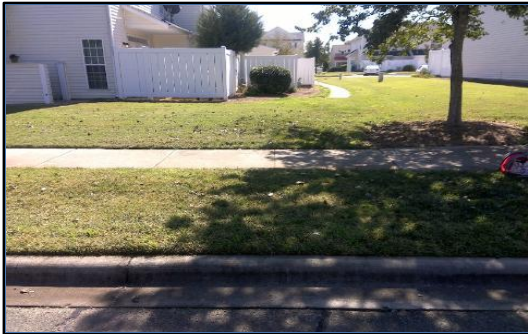
Corner 3 No Ramp (3z)
