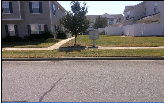
Corner 3 No Ramp (3z)
