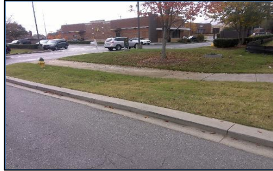
Corner 4 No Ramp (4z)
