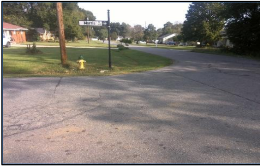
Corner 1 No Ramp (1z)
