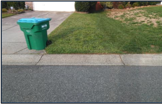
Corner 1 No Ramp (1z)
