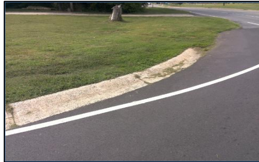
Corner 4 No Ramp (4z)
