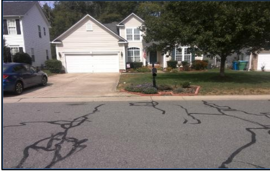
Corner 1 No Ramp (1z)
