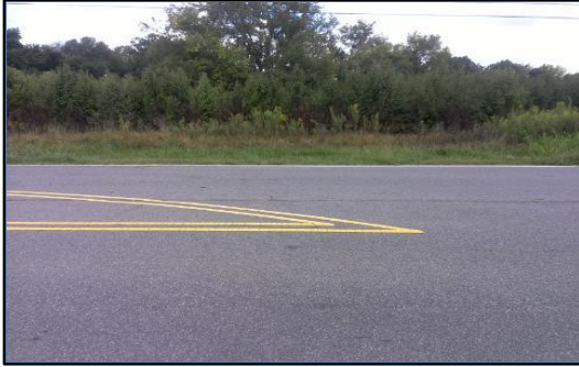
Corner 1 No Ramp (1z)
