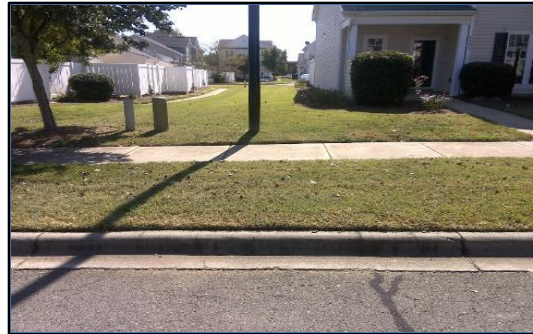
Corner 4 No Ramp (4z)
