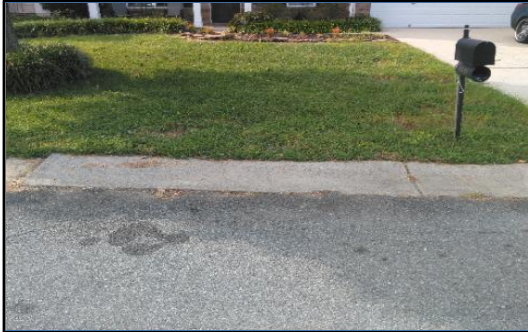
Corner 3 No Ramp (3z)
