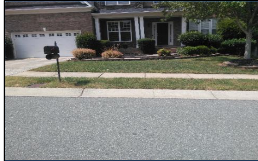
Corner 4 No Ramp (4z)
