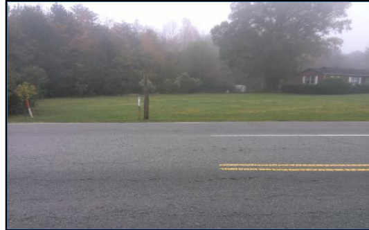
Corner 4 No Ramp (4z)
