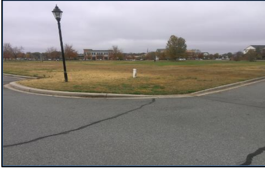
Corner 1 No Ramp (1z)
