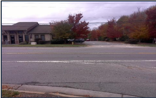
Corner 4 No Ramp (4z)
