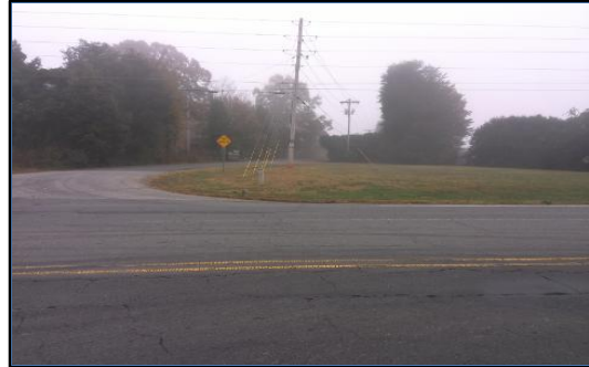
Corner 4 No Ramp (4z)
