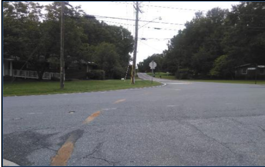
Corner 3 No Ramp (3z)
