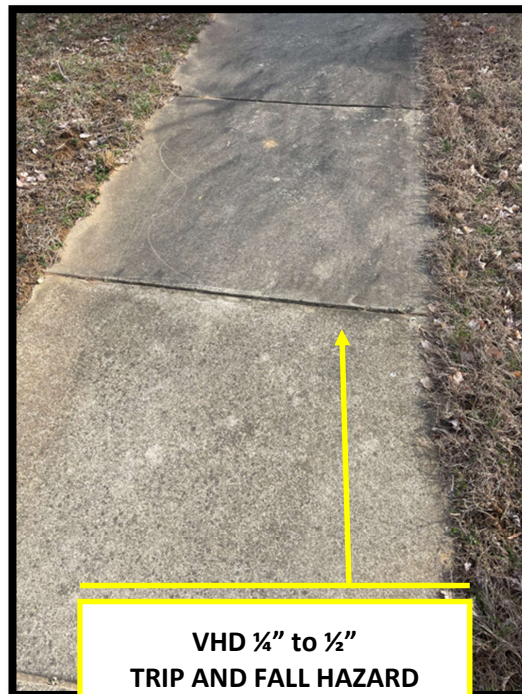
VHD ¼" to ½" TRIP AND FALL HAZARD Repairable using Precision Concrete Cutting Process
